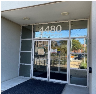
Entrance to 4480 Clayton Building
